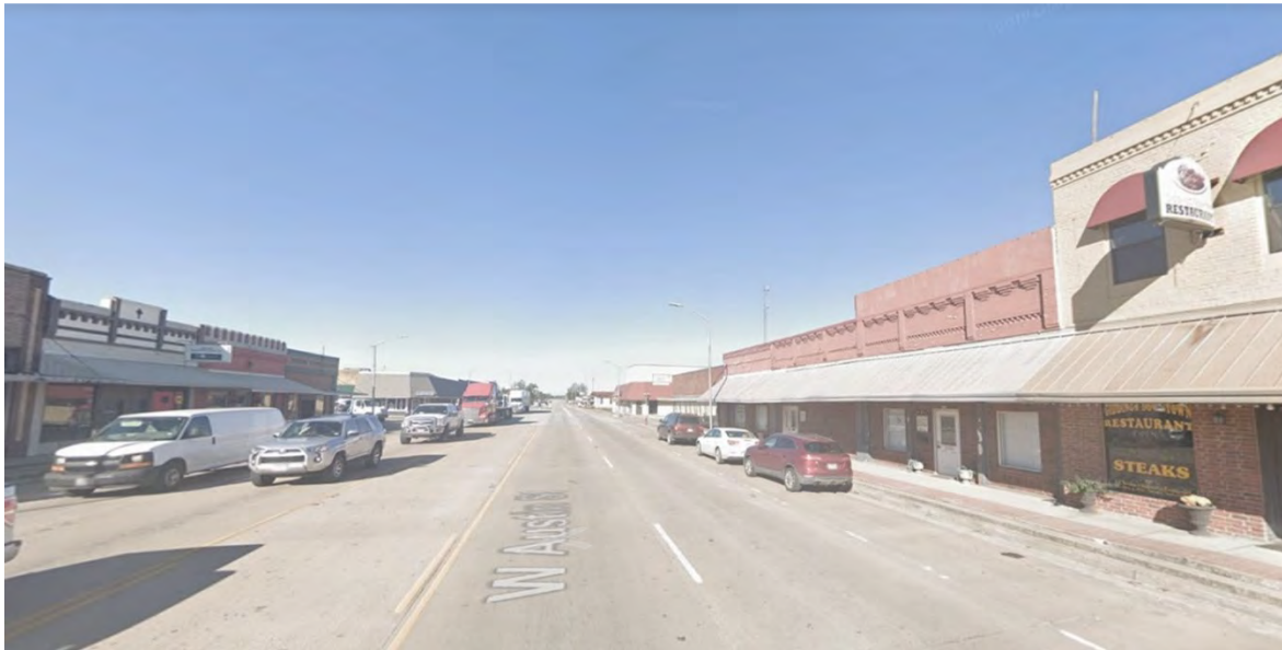
FIGURE 5.4: EXISTING US-290 CONDITION
