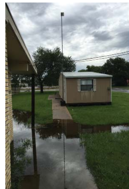
Example of Additional Water Drainage Issues at Site
